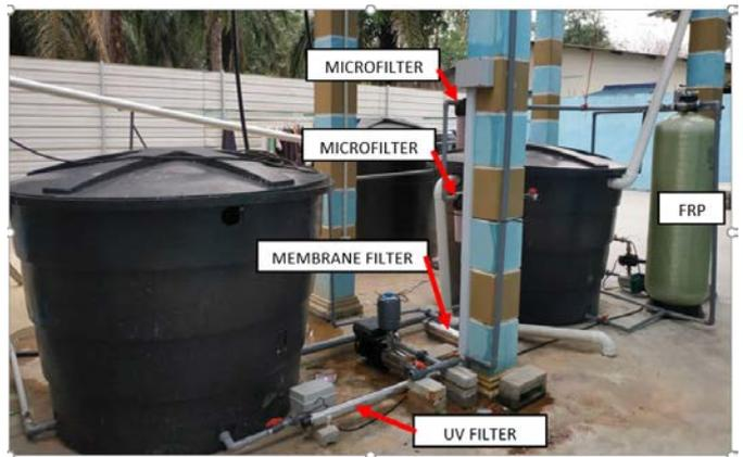
Figure 6: Filtration system for groundwater and rainwater
